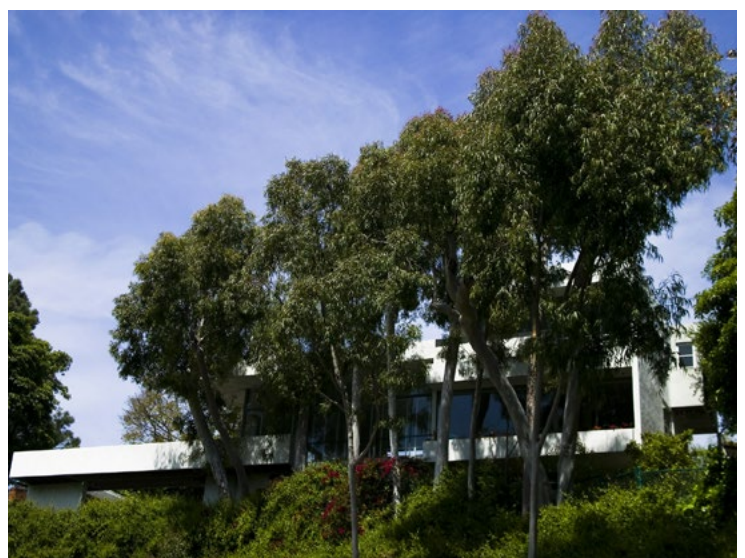
Fitzpatrick Leland House (R. M. Schindler, 1936) © Patricia Parinejad/MAK Center
