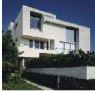
MAK Center for Art and Architecture, Los Angeles Mackey Apartments (R. M. Schindler, 1939), exterior view © Gerald Zugmann/MAK
