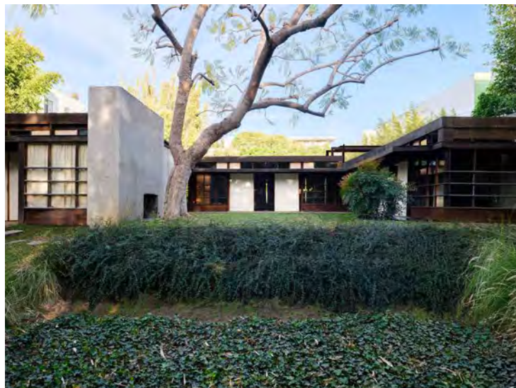
MAK Center for Art and Architecture, Los Angeles Rudolph M. Schindler House (R. M. Schindler, 1921/22), exterior view © Tag Christof
